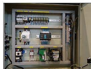
電控系統經由plc可程式控制器，控制系統穩定檢修容易 All operation function are controlled through a programmable logic controller.
